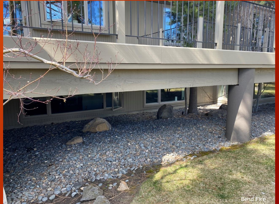
Noncombustible rock under decking
