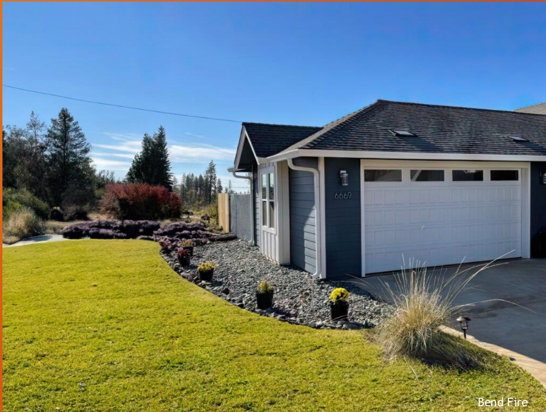
Noncombustible rock around siding
